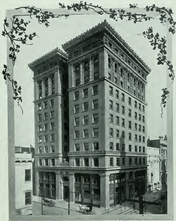
HAYWARD BUILDING. Cor. Montgomery and California Streets
